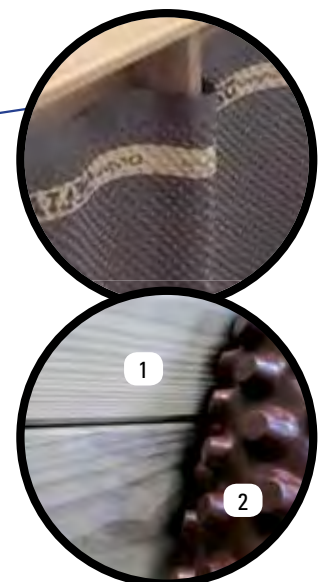
1- Wood frame 2- Roll of alveolar protection and drainage of HDPE
